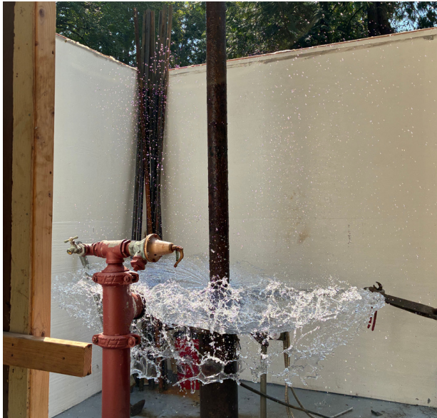
Old pipe being removed from lower section.
